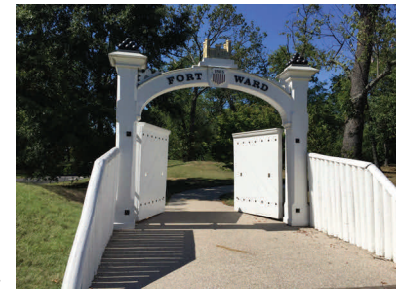
Reconstructed ceremonial Fort Ward Gate
