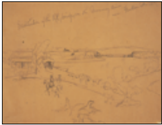
Destruction of the RR bridge over the Monocacy River
