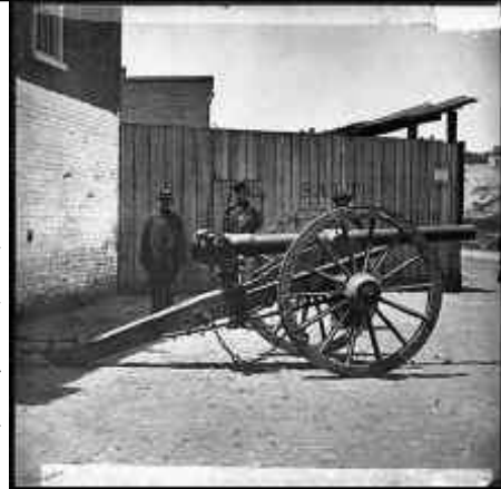
12-pounder Whitworth rifled cannon and projectile.
